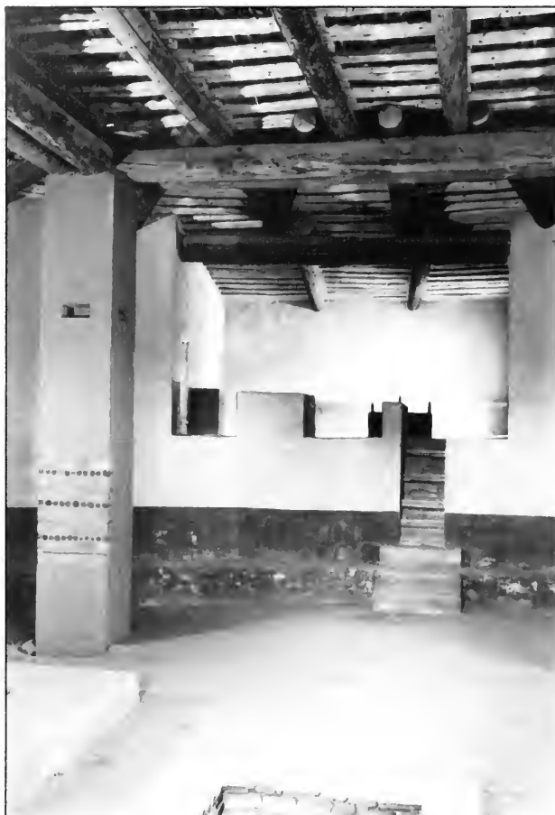
Figure 7.11. Interior of restored Great Kiva, looking toward north altar room. Crossbedded poles in roof support column left exposed to demonstrate method of construction.
